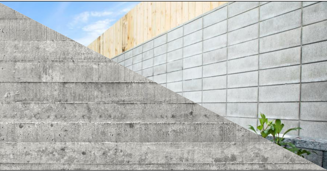
RETAINING WALL - KEYSTONE BLOCK + SHUTTER
