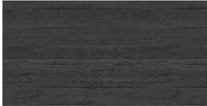
BLACK OXIDE CONCRETE TILT SLAB WALL
